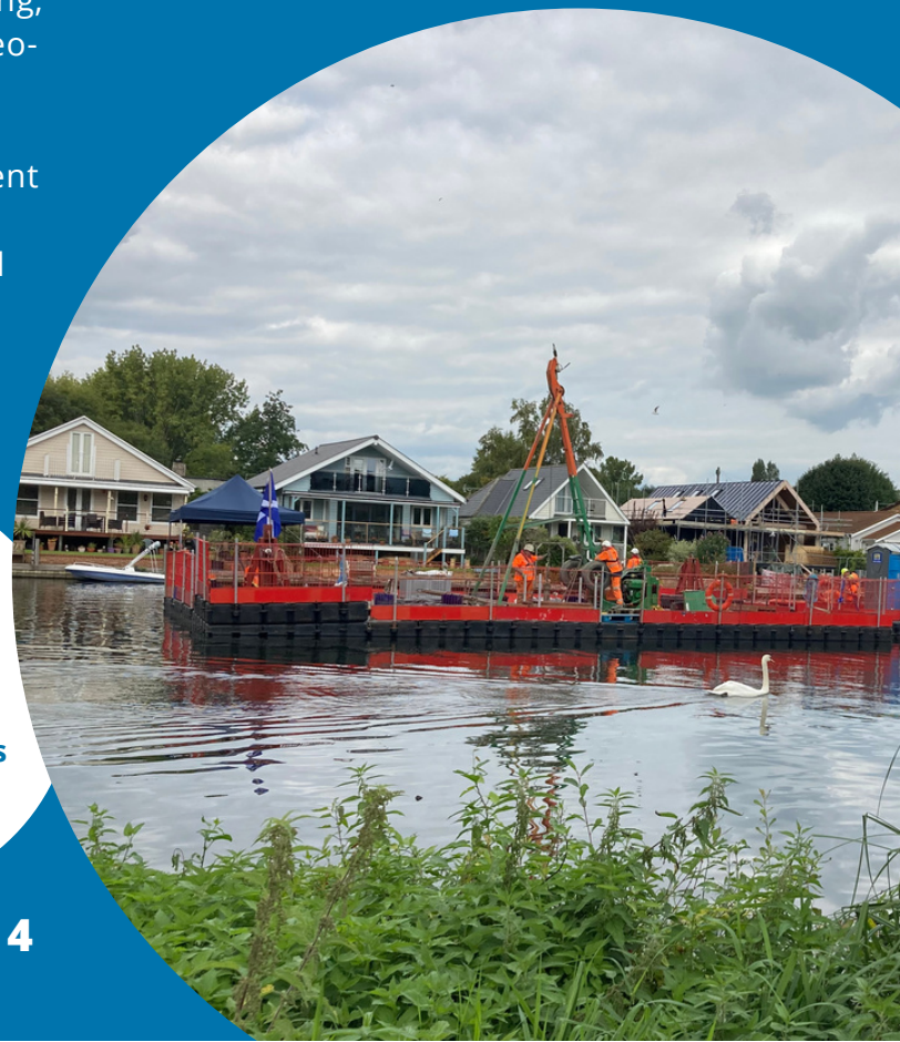
Cable percussion rig on a pontoon at Walton on Thames
