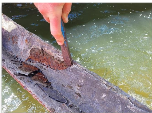
Much of the weir's structure is now suffering corrosion
